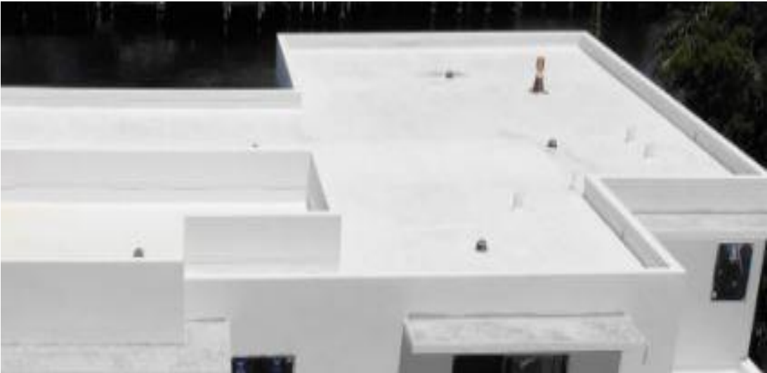
ROOFING – 60# TPO MEMBRANE OVER ¼” DENSDECK ROOF BOARD
