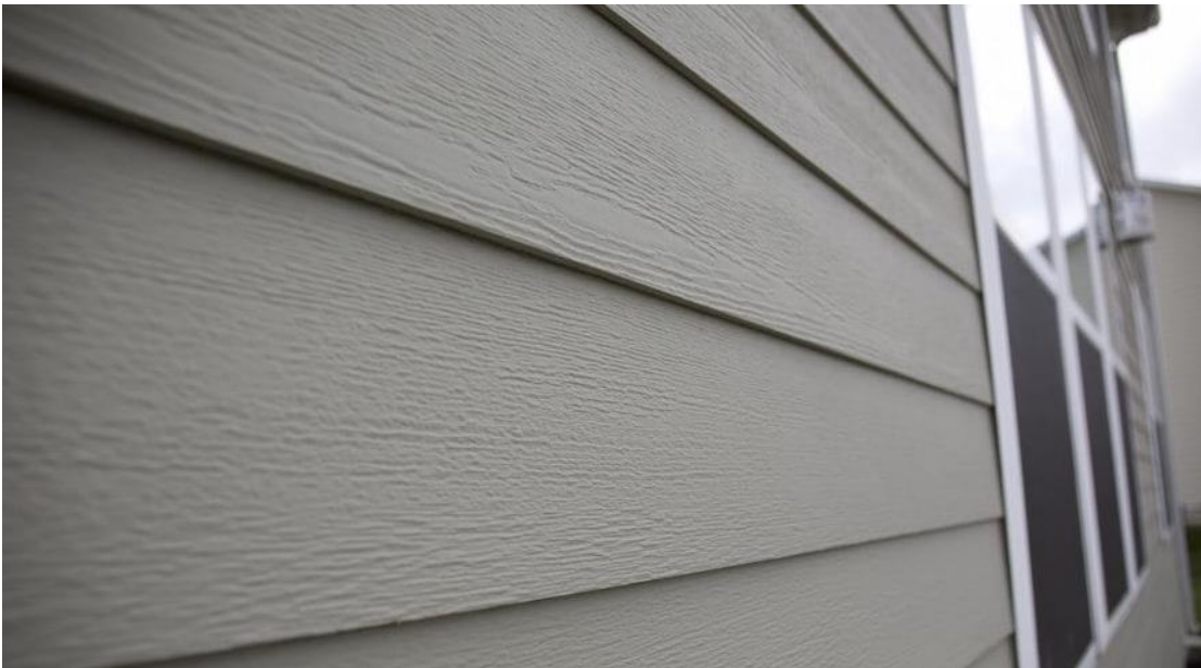
SIDING – JAMES HARDIE: CEMENTITIOUS LAP SIDING OVER 30# ORGANIC FELT UNDERLAYMENT. COLOR: LIGHT MIST
