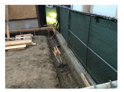
The third photo is looking in a southeasterly direction towards what was the east exterior wall of the previous garage which is completely gone / demolished. The wood form boards are for the <u>new</u> east wall.
