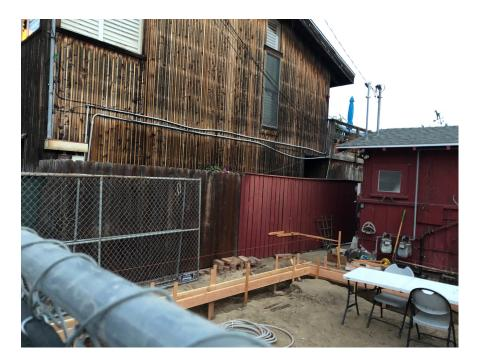
The fourth photo is looking south towards the eastern portion of what was the south exterior wall of the previous garage which is completely gone / demolished. The wood form boards are for the <u>new</u> south wall.
