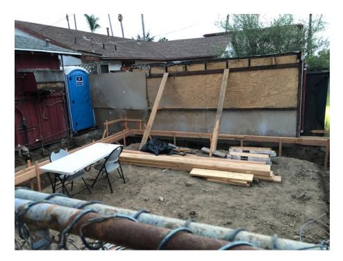
The previously existing North, East and South walls, more than 75 percent of the previous garage walls, have been completely demolished, with less than 25 percent of the prior exterior walls remaining today. The demolition has exceeded that allowed for CDP exemption.
