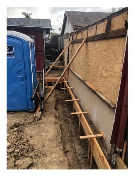
In the foreground on the right side of the above photo is what little remains of the previous west wall of the previous garage. Plywood was applied to what was the exterior face of what little wood wall framing remains. The high cripple wall studs and the top plate and bottom plates that might have previously existed are now gone / removed.
