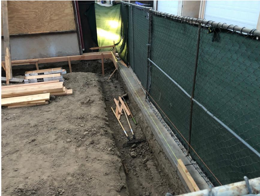
The third photo is looking in a southeasterly direction towards what was the east exterior wall of the previous garage which is completely gone / demolished. The wood form boards are for the new east wall.
