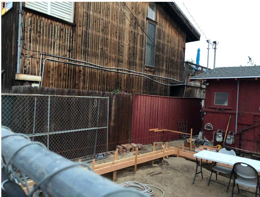
The fourth photo is looking south towards the eastern portion of what was the south exterior wall of the previous garage which is completely gone / demolished. The wood form boards are for the new south wall.
