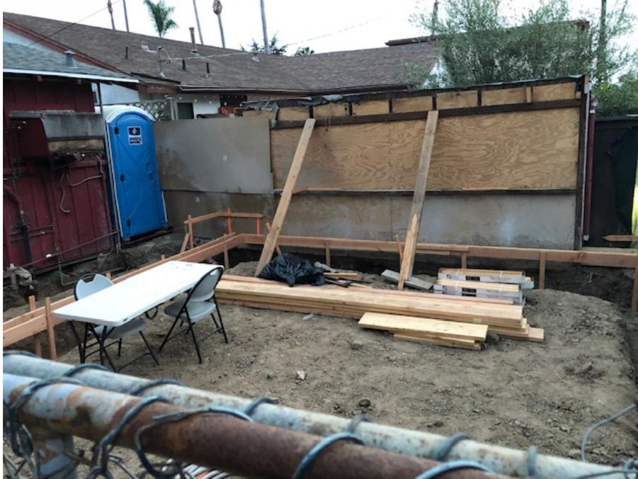
The previously existing North, East and South walls, more than 75 percent of the previous garage walls, have been completely demolished, with less than 25 percent of the prior exterior walls remaining today. The demolition has exceeded that allowed for CDP exemption.
