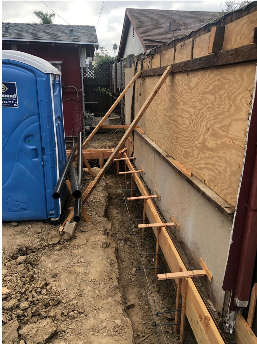
In the foreground on the right side of the above photo is what little remains of the previous west wall of the previous garage. Plywood was applied to what was the exterior face of what little wood wall framing remains. The high cripple wall studs and the top plate and bottom plates that might have previously existed are now gone / removed.
