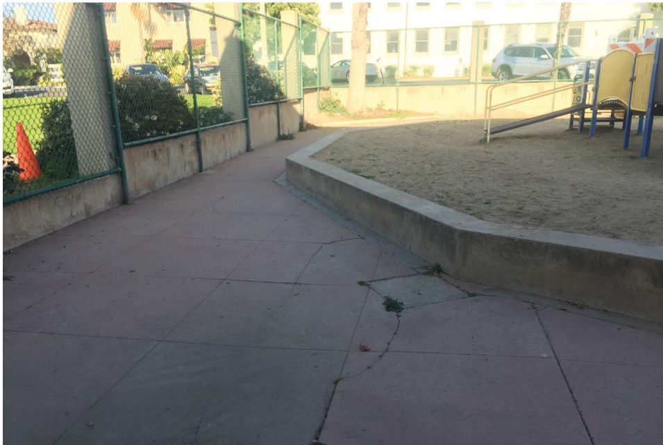
LA JOLLA REC CENTER RENOVATION EXISTING CONDITIONS
