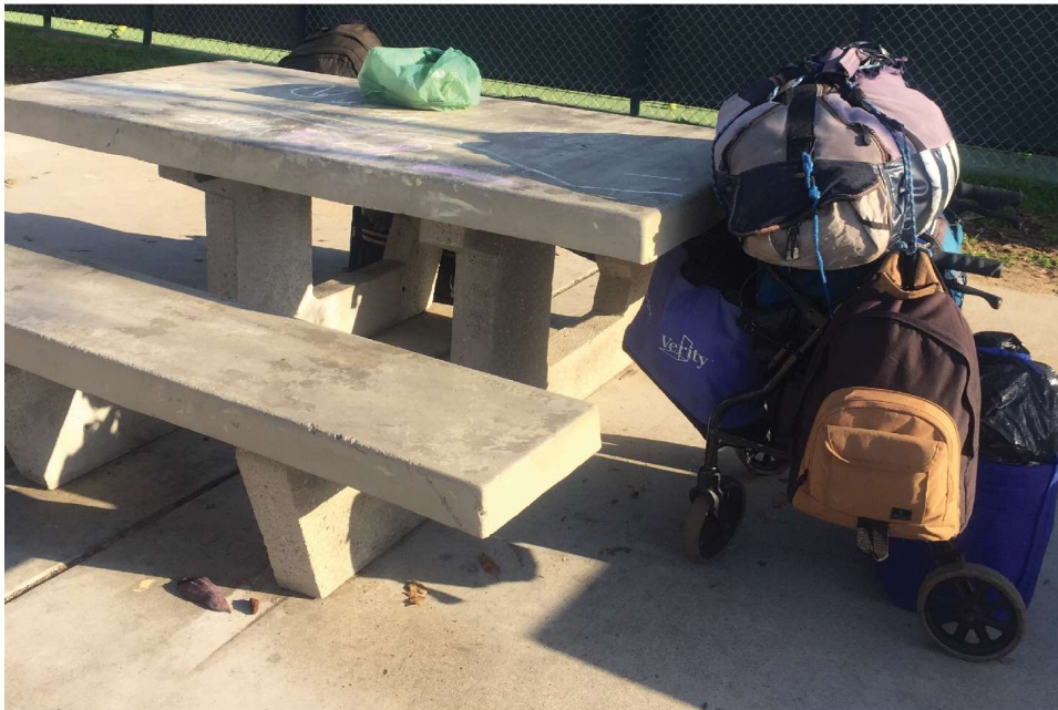
LA JOLLA REC CENTER RENOVATION EXISTING CONDITIONS
