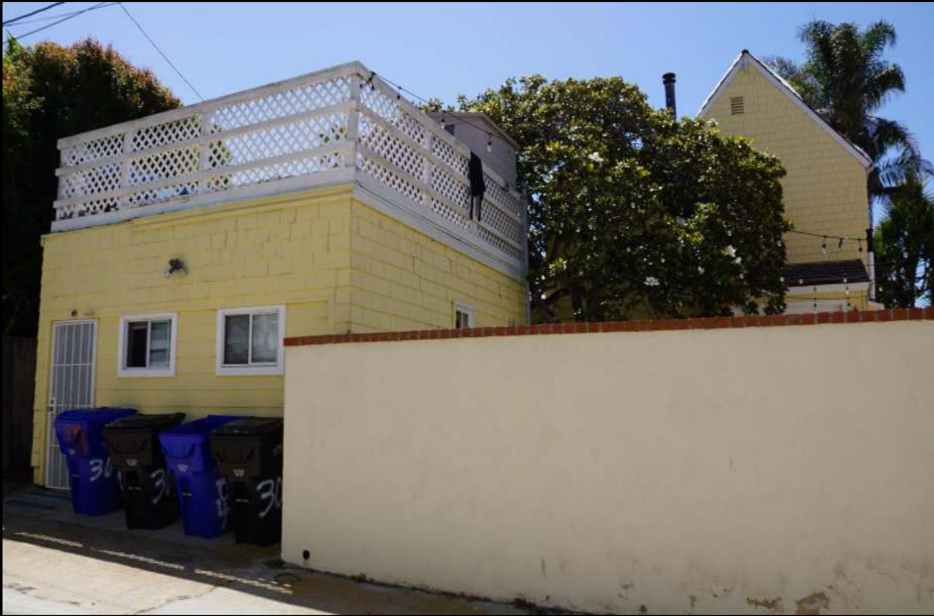
EXISTING 2 ND UNIT – UNPERMITTED GARAGE CONVERSION
