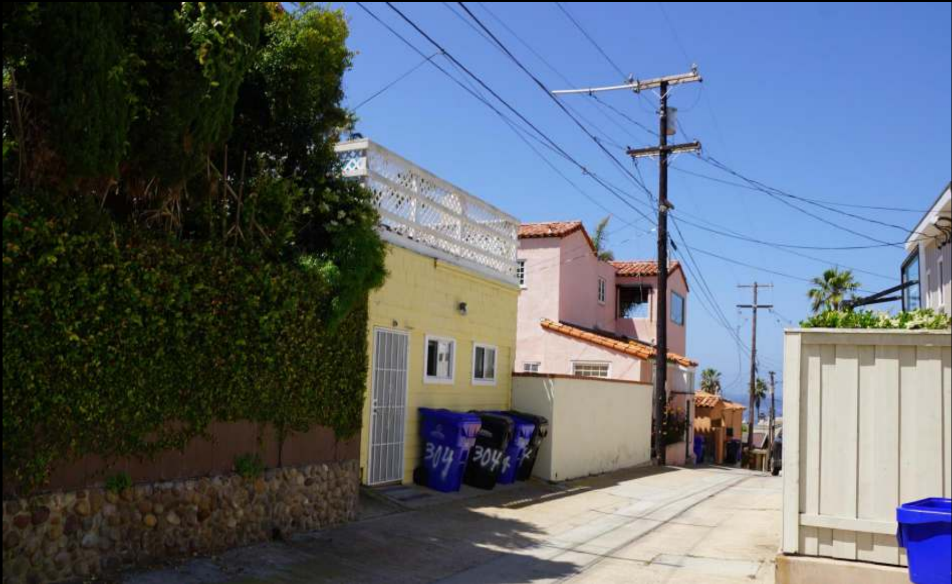
EXISTING 2 ND UNIT – UNPERMITTED GARAGE CONVERSION
